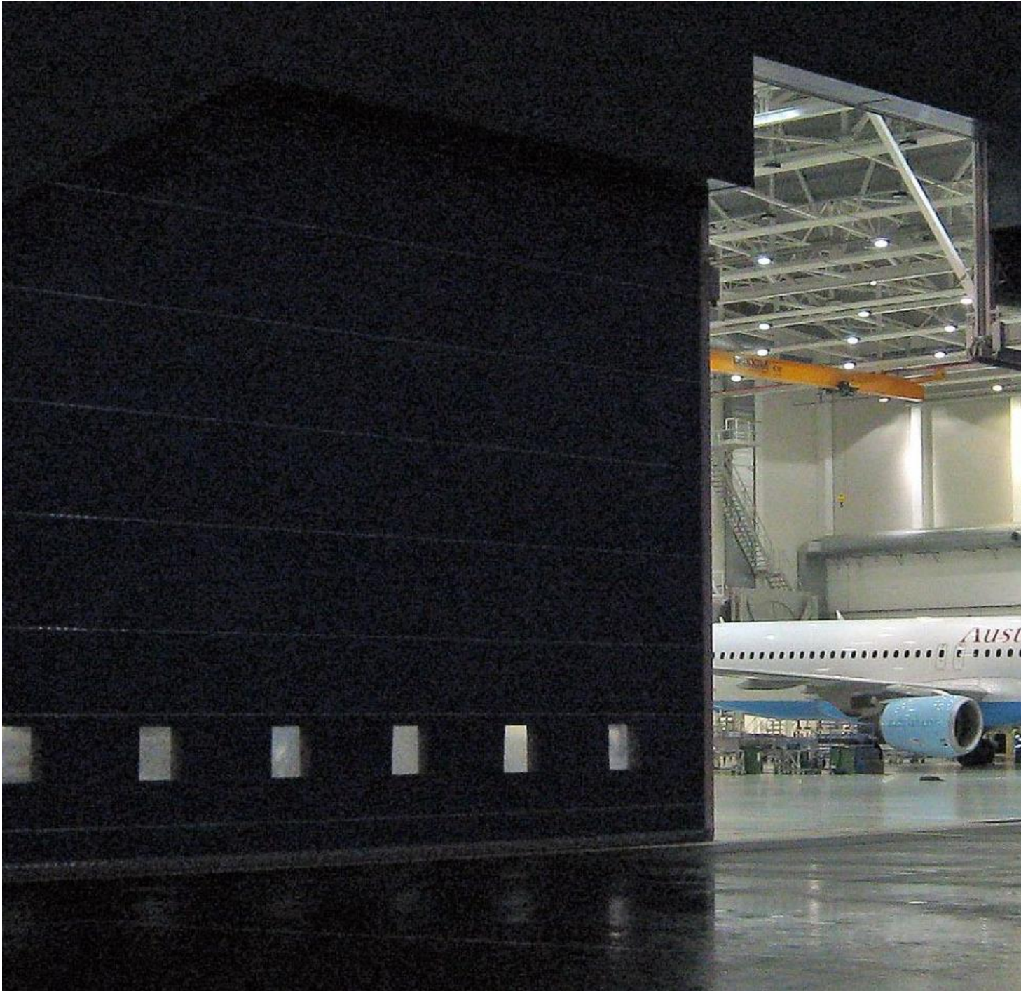
Magnetic MRO hangar in Tallinn
