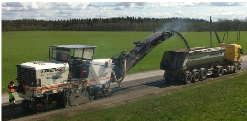
TREV-2 road construction
